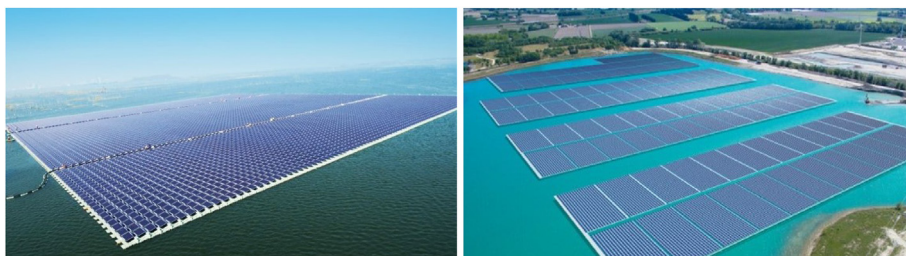
Fig. 1. Floating Solar PV installed on a water body ([31:32]).
