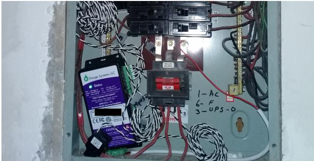
**Figure 3: Smart meter installed in one of the selected households**
